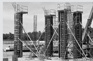
Column Formwork
