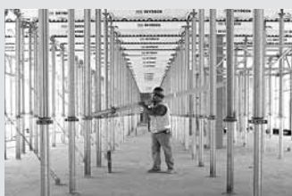
Slab Formwork
