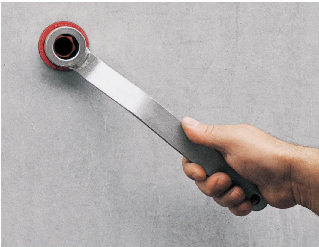
Removing the DK Sealing Cone with the DK Cone Spanner UNI.
