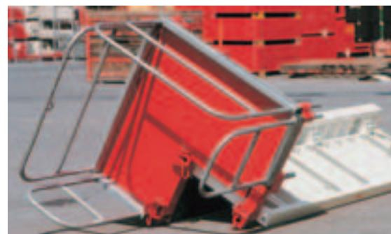
The concreting platform is assembled on column halves whilst in a lying position.
