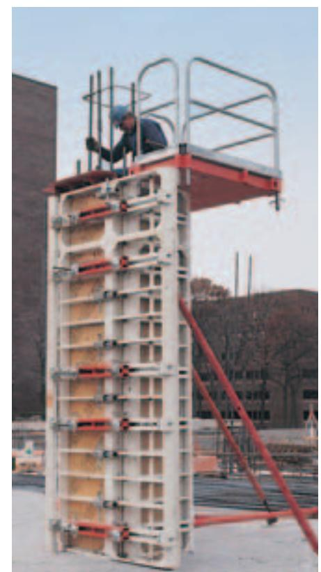
Oversized RAPID Column Formwork stiffened with steel waler SRZ.
