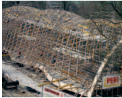
MULTIPROP Props carried the timber construction and facilitated the curved shape of the gridshell.
