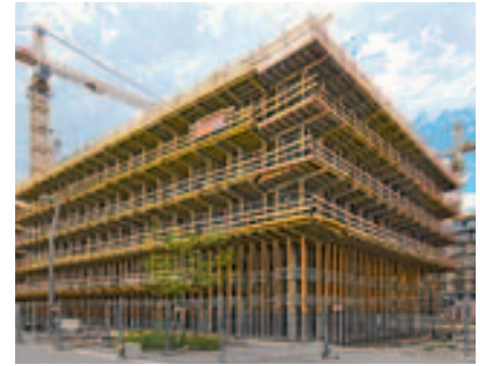
The PERI solution with MULTIPROP and MULTIFLEX, as well as for forming the circumferential balconies, served simultaneously as working scaffold.
