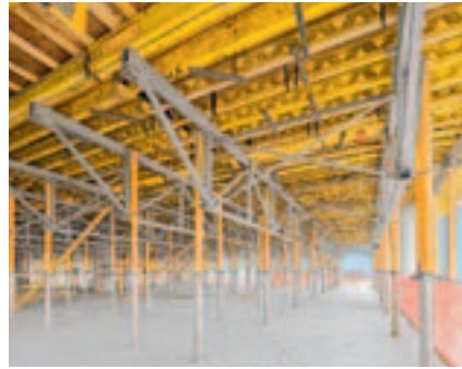
MULTIPROP Props, used for large-sized SKYTABLE Slab Tables, facilitate faster cycles with a higher level of safety.
