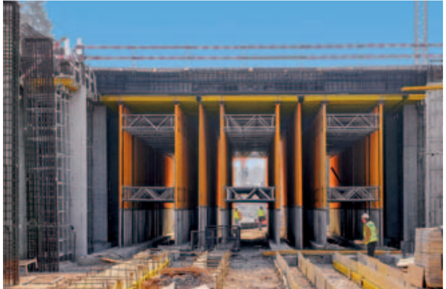
Especially with large slab heights, MULTIPROP Shoring Towers are a cost-effective alternative to standard spatial load-bearing scaffold.
