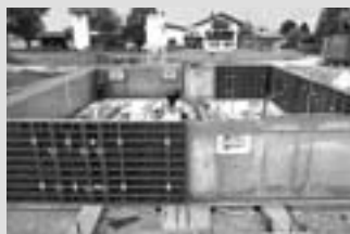
Wall Formwork
