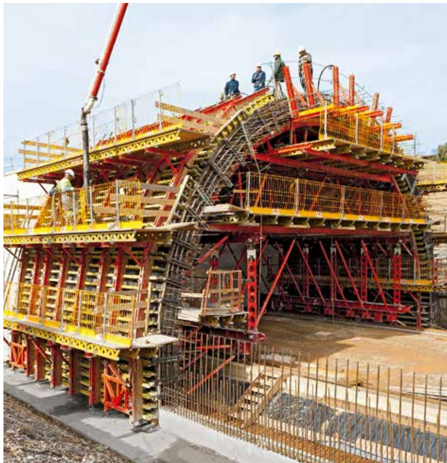
PROKIT EP 110 provides protection on all open edges of the working platforms of this tunnel formwork
