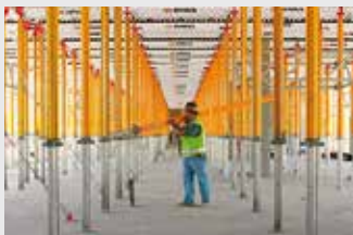
Slab Formwork
