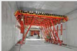
Tunnel Formwork
