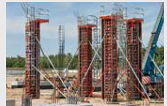
Column Formwork
