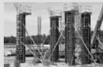
Column Formwork
