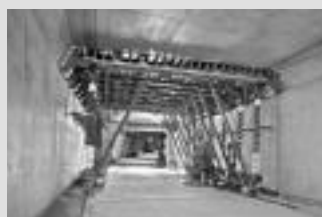
Tunnel Formwork
