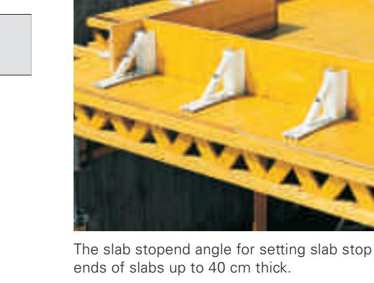
The slab stopend angle for setting slab stop ends of slabs up to 40 cm thick.
